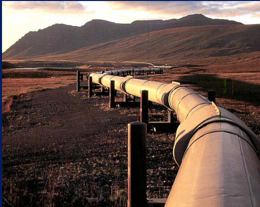
Figure 1: A real-life pipeline.
